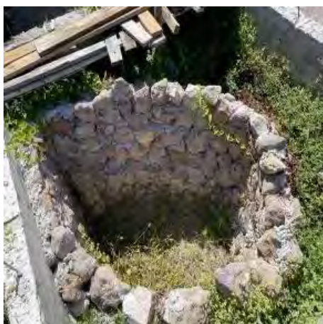
Figure 6.4 Cesspit in construction (VEI, 2023)
